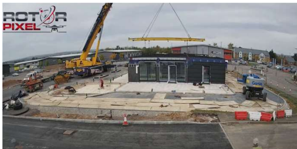
Final module of ground floor installed
