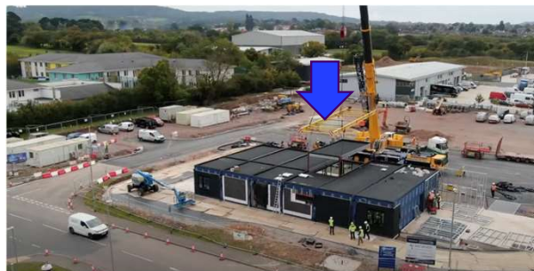
Ground floor finished, modular roof now installed
