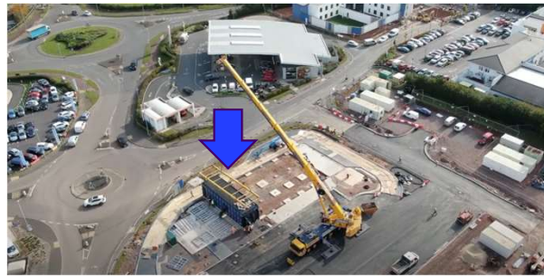
Ground floor finished, modular roof now installed
