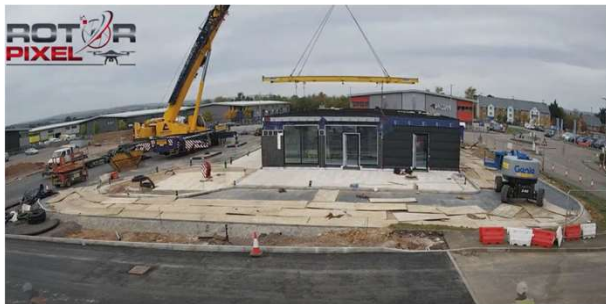
Final module of ground floor installed
