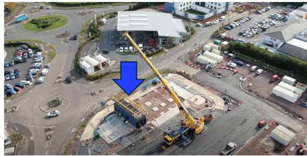
Ground floor finished, modular roof now installed
