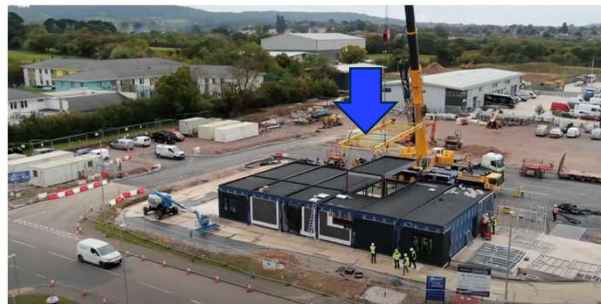
Ground floor finished, modular roof now installed
